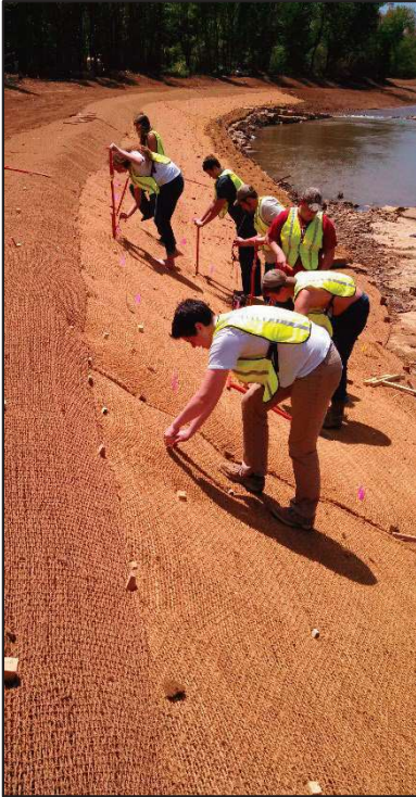
Geotextiles allow for plants to grow while keeping the soil in place. (Photo by Ben Thompson)
